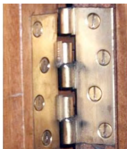
Hinges on high traffic areas which have become badly worn
