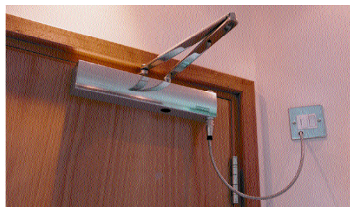
Electro-hydraulic hold open door closer
