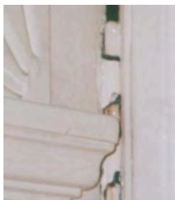
Hinges on high traffic areas which have become badly worn
